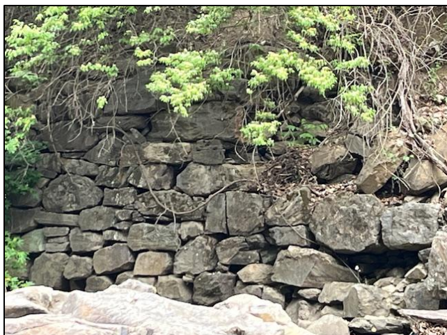
Figure 14 —Stones quarried from the Indian Run bedrock make up the roadbed for the historic Washington and Old Dominion Railroad, a prime example of 19 th -century engineering, visible at Huffman's Falls.
